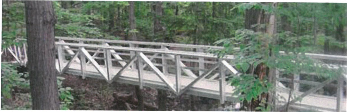
Figure 2. Footbridge on the Rensselaer Technology Park property.
