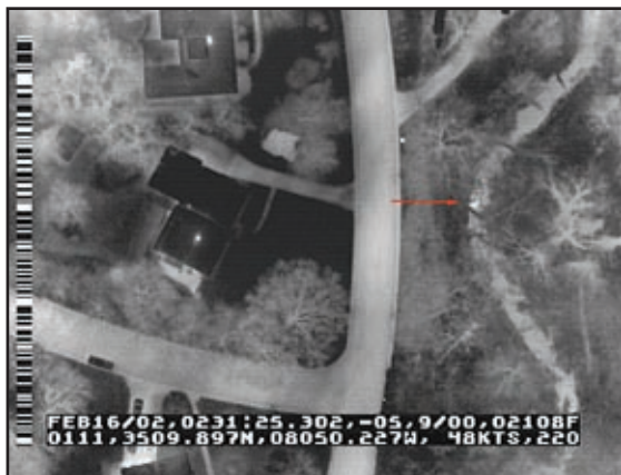
Figure 72: Aerial thermography showing sewage leak
